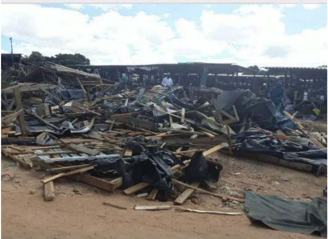
Figure 1: Market sheds being demolished by the City Council.
